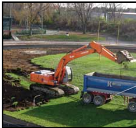
Excavating of Matt Senffner Field began in mid-November.
